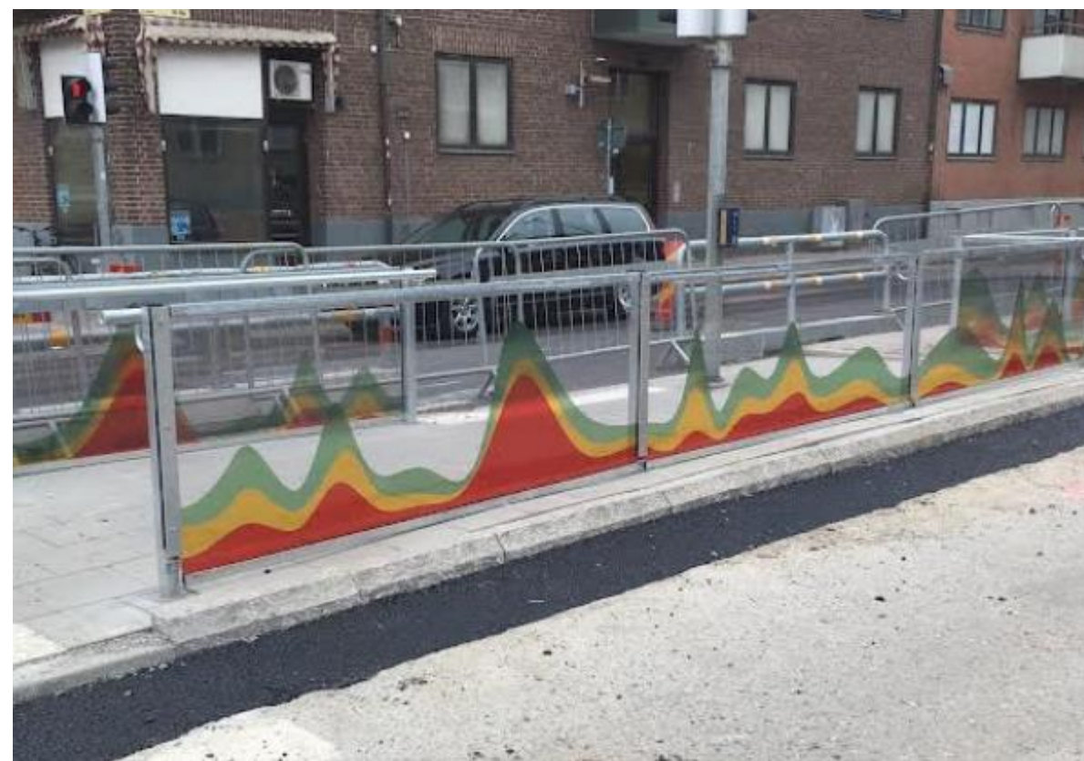
Digital print: Single coat, Laminated Hammerglass 6 mm + 6 mm. End result; "Double coated" Hammerglass
